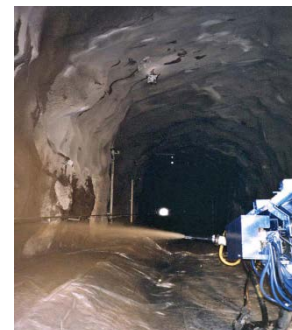
PENETRON® ADMIX ENHANCED SHOTCRETE – PAES™ APPLIED IN RAILWAY TUNNEL PROJECT IN SWEDEN
