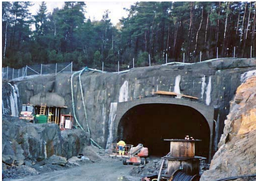
SWEDISH WEST COAST RAILWAY ÅSA TUNNEL 4000 M 2 SLURRY PROOFED ROOF AREA
