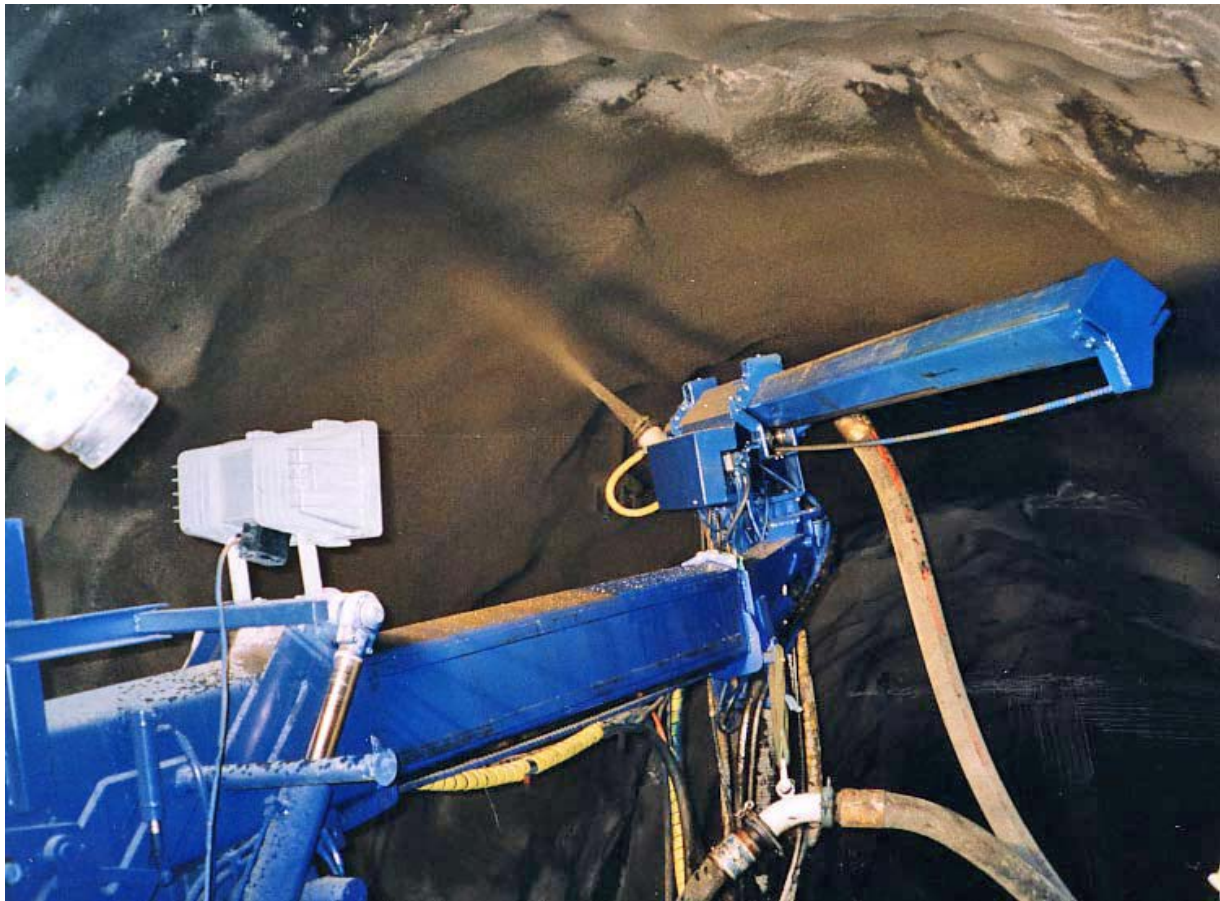
PENETRON® ADMIX Shotcrete BOTNIA Railway tunnels in Sweden
